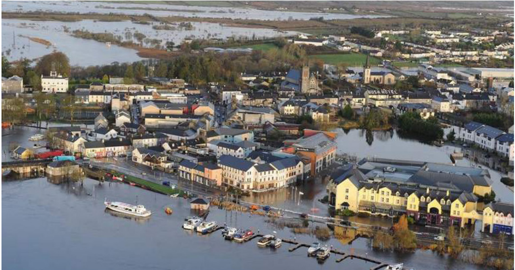
Figure 1: Flooding in Carrick-on-Shannon, Co. Leitrim in November 2009
