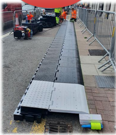
Modular Paving Under Construction
